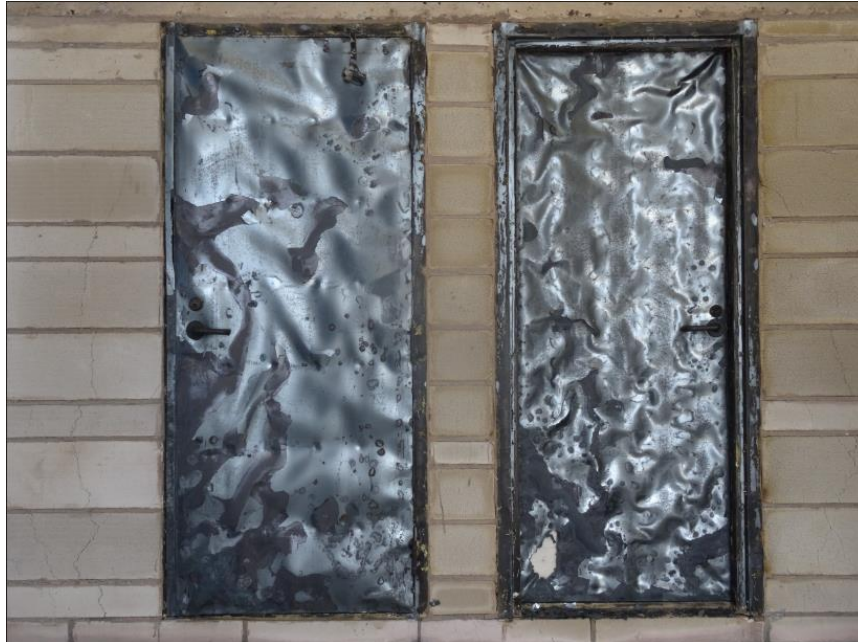
Fig. 6 Exposed Side after test
