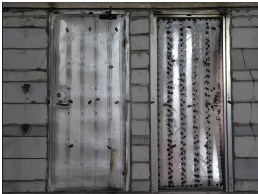
Fig. 4 Unexposed Side after 180 Minutes
