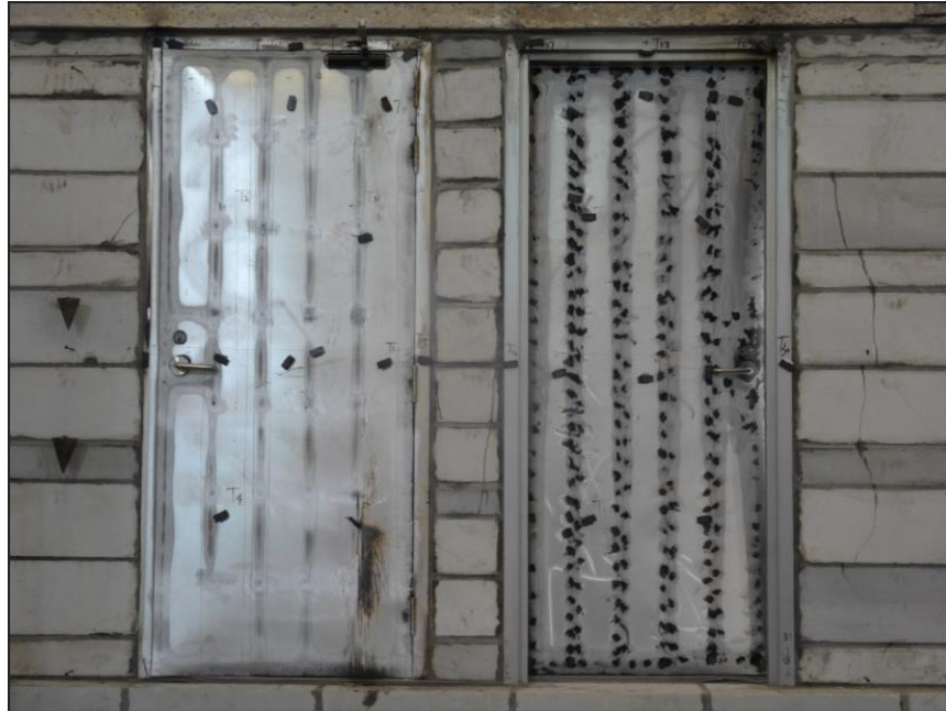
Fig. 3 Unexposed Side after 120 Minutes
