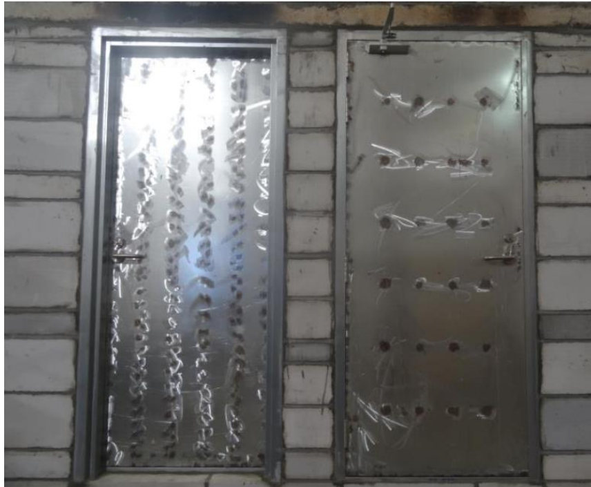
Fig. 1 Exposed Side Prior to the Fire Test
